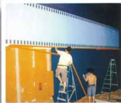
Acoustic Project at King's Theater, Sarawak House Shopping Complex.
